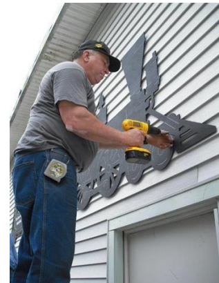
Tom Coulombe Installing Train Sign At the Club
