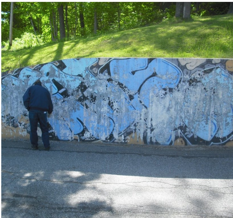
Power washing needs to be completed before the wall is repainted
